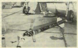
UNLOADED? After removing two 275-gallon tanks from an F-100 one of the maintenance men noticed that the push-away pin for special weapons stores on the left intermediate station was extended. He tried unsuccessfully to retract it by pushing it in with his hands. He then decided to do the job electrically and ther made a too quick check of the left pylon to see at it was not armed with cartridges or failed to
